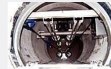
These facilities are being used nationwide as a new armor for small-scale contaminated-water-transferring pumping stations, which are essential to spread the use of sewerage systems. The facilities are compact, with a tank to collect contaminated water (manhole) set with an underwater pump and employed in places with insufficient space for other facilities.
